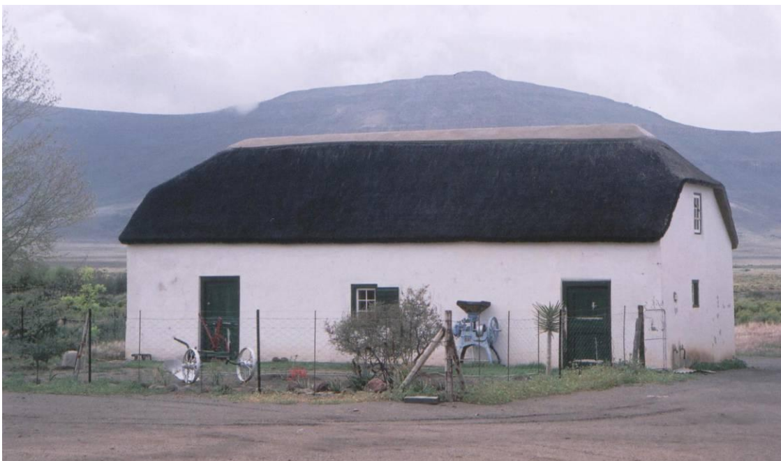
Figure 4 The thatched two-roomed cottage was restored in 2004 but without the hearth and chimney stack projecting from the kitchen end. (AP 2006)
