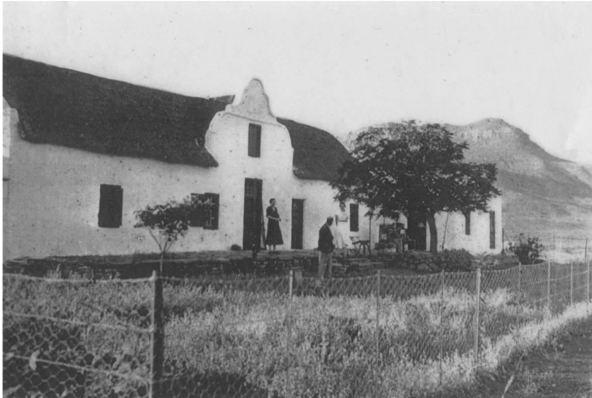
Figure 5. In the early 1800s a third (T-plan) house was built. The doors, windows, ceilings, beams, etc. were of cedar wood. The gable, in the Prince Albert style, was probably added later. The stoepkamer was also a later addition. It was completely gutted by fire in 1949. Note the door next to the front entrance. According to Jacoba de Villiers (born van der Merwe), Carel and Katie van der Merwe feature in this photograph taken in about 1937.
