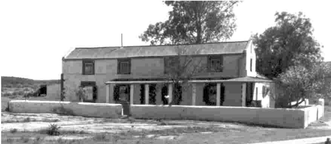
*Figure 7(b): L-shaped double-storey house (building no.7) with corrugated iron roof, verandah and stone walf wall (c1874). Imported Oregon pine was used throughout. “The Manakwalanders” was filmed here.*
