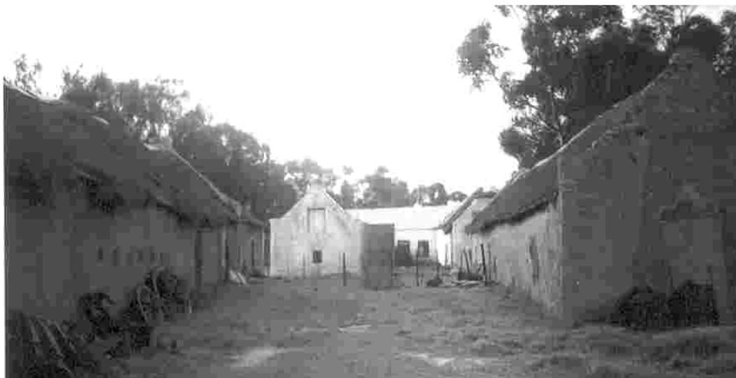
*Figure 12. Parallel outbuildings (nos.4 and 5) of clay and raw bricks, photographed by the writer Karel Schoeman in June 1986. Building no.4, which also housed a two-roomed cottage with outside hearth, was demolished in 1996 after heavy rain caused walls to collapse.*
