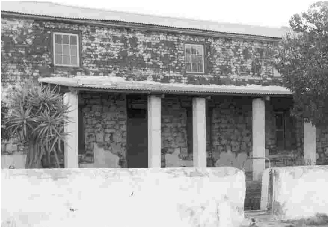
*Figure 8. When re-plastering the double storey house in February and March 2000 it was discovered that the walls of the lower section were of dressed stone.*
