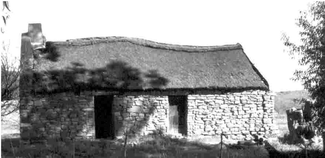
*Figure 9. A rectangular thatched two-roomed un-plastered stone cottage with internal hearth (building no.13). There is evidence of a foundation to its right - a buitekamer or a stable?*
