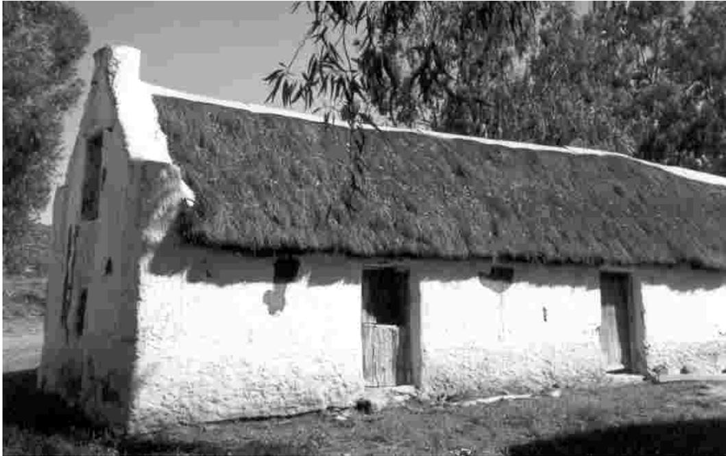
*Figure 13. Rectangular outbuilding thatched with zonkwariet (building no.3), having cedar wood doors and reed ceilings in the two rooms on the left. Roof construction has a steep pitch to facilitate drainage of the thatch.*
