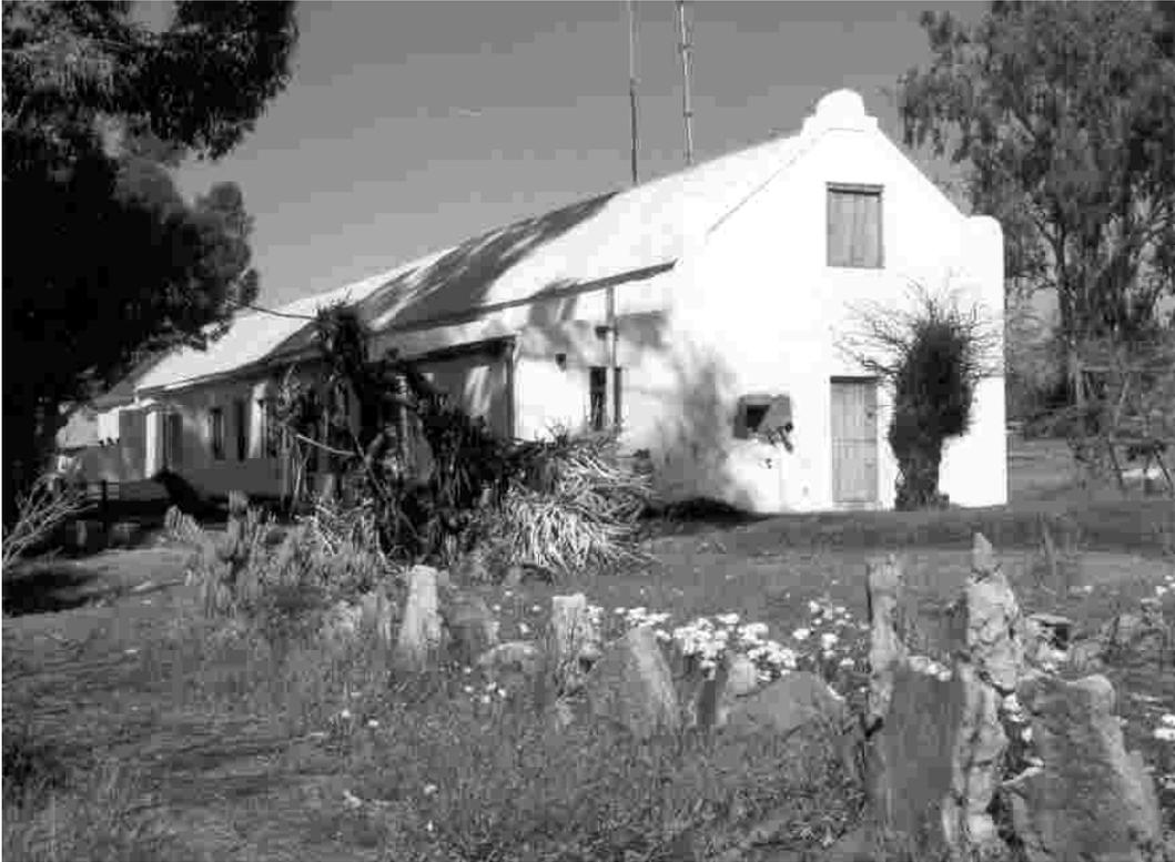
*Figure 4. The 44 metre long front façade of the T-shaped main homestead, built c1874 (building no.1), with enclosed verandah and new double garage on the left, plus an adjoining thatched cottage on the extreme left (building no.2) with stable door and shuttered window (see Fig.6).*
