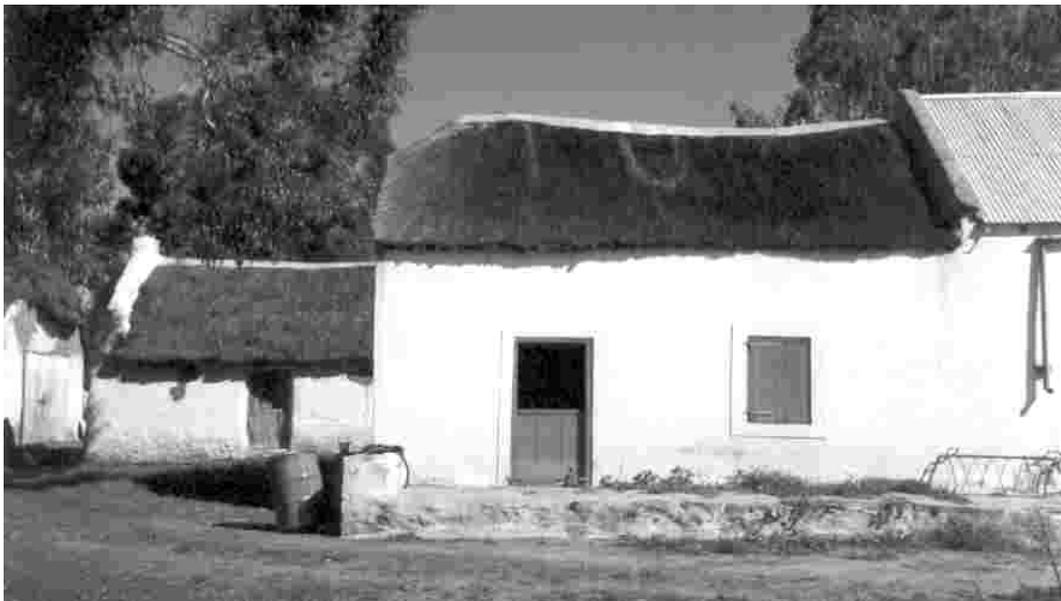
*Figure 6. Thatched cottage (building no.2) with stable door and shuttered window that abuts the main dwelling. The cottage retains its reed ceiling but sacrificed the kitchen and hearth in 1970. In February 2000 the roof collapsed and it has now, regrettably, been replaced with corrugated iron. In the background is an outbuilding housing slag- and tuiekamers (building no.3).*
