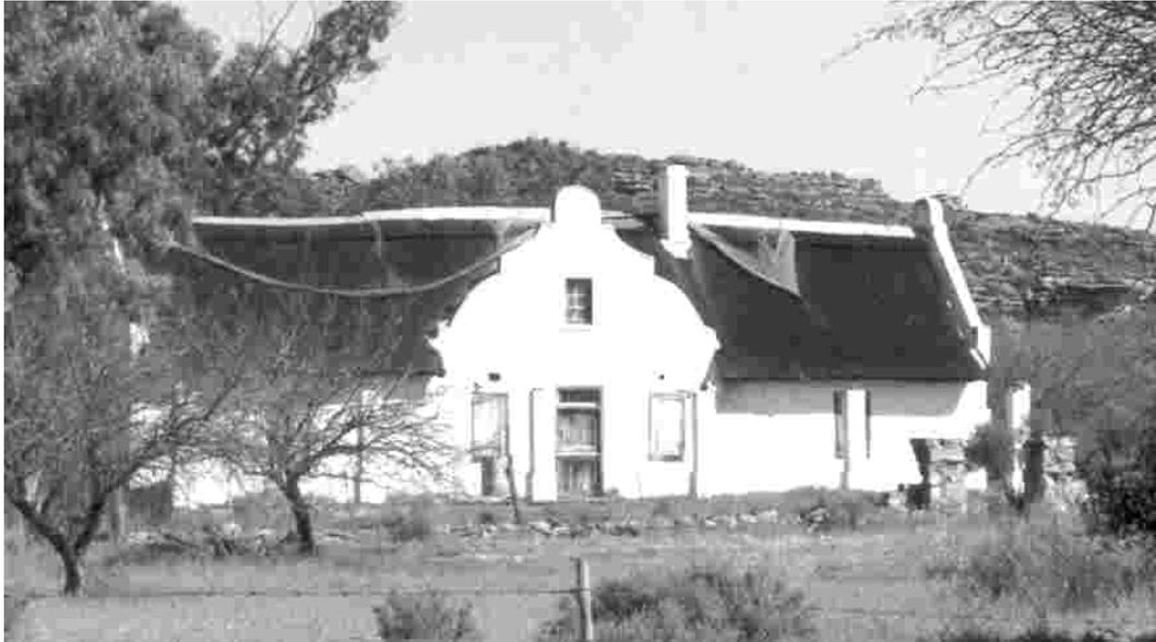
*Figure 10. Lokenburg's third homestead (building no.14). A T-plan with Cape Dutch style gable added during 'restoration' in 1956. The voorkamer, two bedrooms, dining room and passage all had reed ceilings, which were replaced with new beams and fresh reeds in 1956. The thatch is springbokriet, which is superior to zonkwariet. This is where the Laurences lived from 1911 until 1978.*
