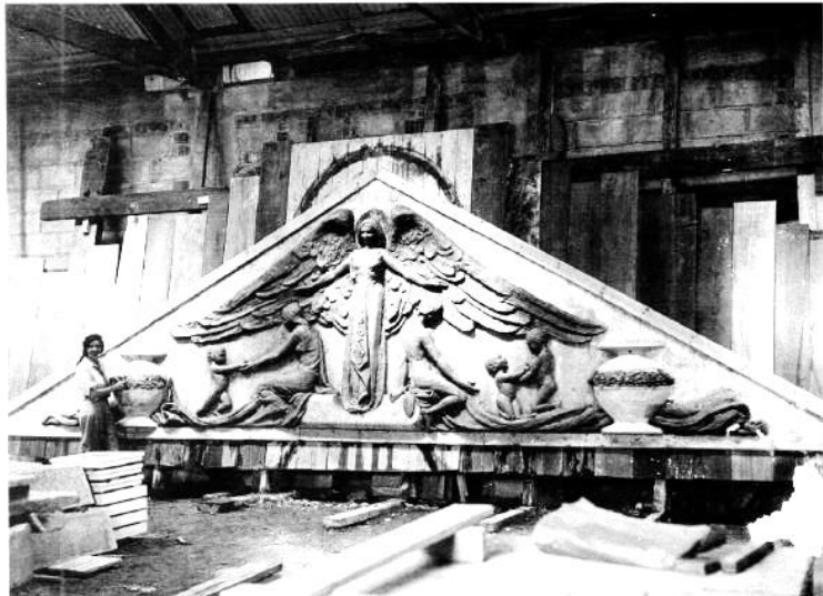
Fig. 4.52: Wynne at Salt River Cement Works with the sculpture to adorn the pediment of the Women's Wing.
