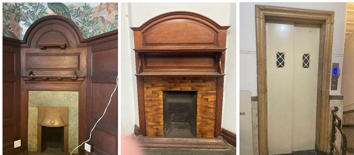
Left & Centre: Period fire surrounds. Right: Lift doors.
