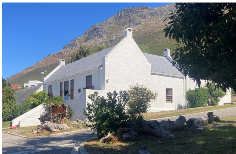
Oatlands 'Commandants House' restored 1975 after being gutted by a mountain fire on Christmas Day 1972 (photo © John Kramer 2026).
