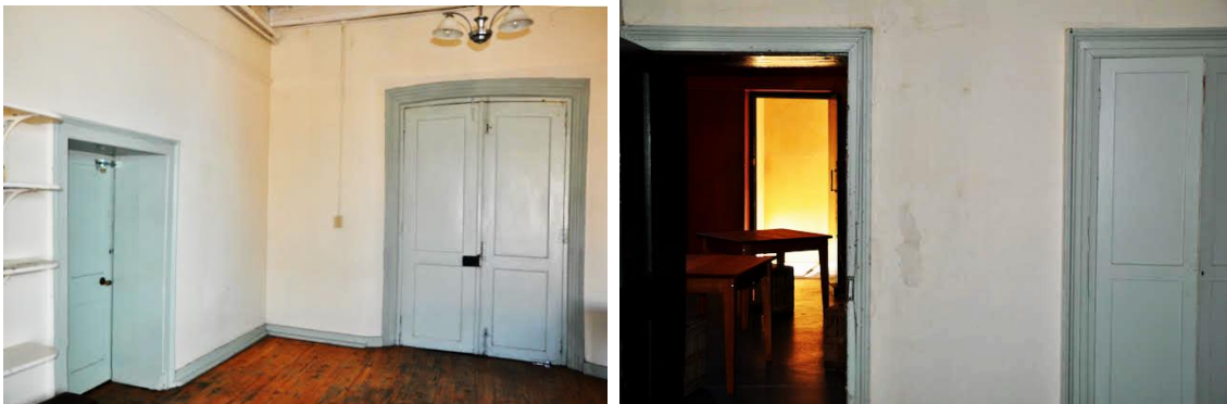
Interior of the dwelling.
