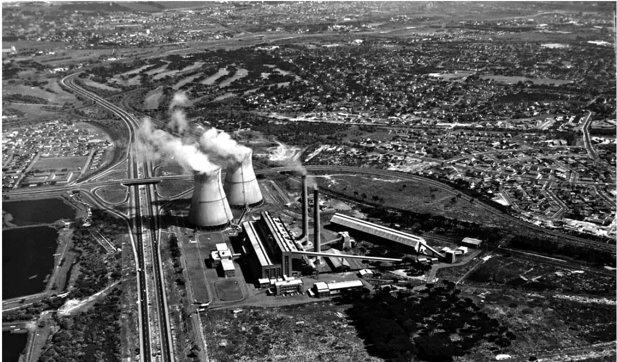
Athlone power station cooling towers in the 1960s (posted by Harry Valentine Cape Historical Society). The brick chimneys are 99 metres high.
