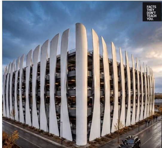
Recycled wind turbine blades converted to clad a parking garage.
